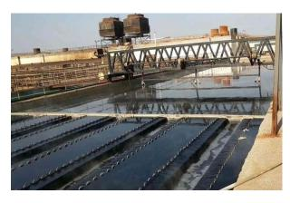
hydraulic reciprocating rectangular tank bottom scraper has the characteristics of less moving parts, less maintenance, continuous sludge transportation, high reliability, simple installation and sludge concentration. WF bottom scraper has been successfully applied to a large number of different types of sludge sedimentation systems with a wide range of applications.
